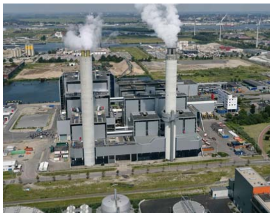
Figure 1. Aerial view of AEB. The left stack is the new Waste Fired Power Plant, the right stack is the existing Waste to Energy plant, the sludge digesters from the municipal waste water treatment can be seen in the forefront.
