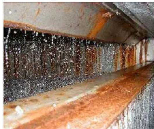
*Figure 2. Corrosion damage to the air supply channel of a large auditorium by LiCl solution aerosol*
