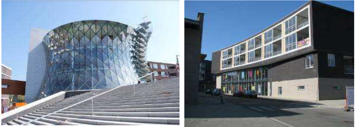
Figure 3 Heerlerheide Centre, cultural building with energy station, school and apartments
