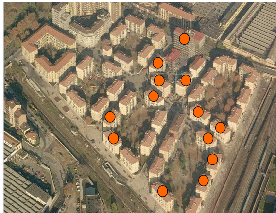
Fig. 3 Arquata district and ATC building PV panels
