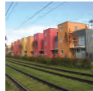
13 Ostfildern, Stuttgart. The new high energy efficient district, heated by the biomass plant
