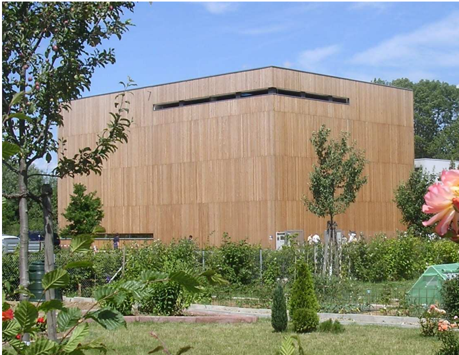
Fig. 1 View on the biomass power plant
