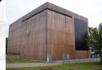
Biomass cogeneration unit 35 kWp
