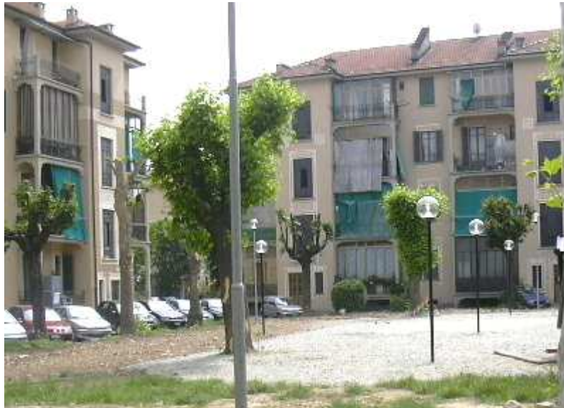
Figure 5 – Internal courtyards lamps
